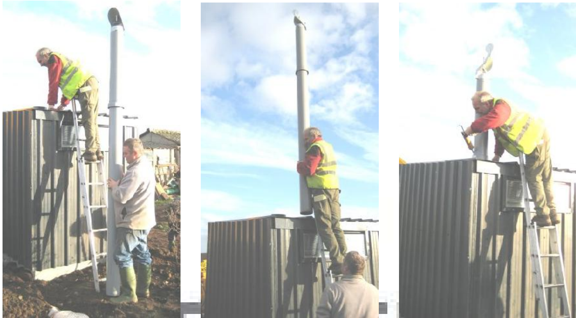
These pictures show a metal building but fitting the vent pipe is the same.
