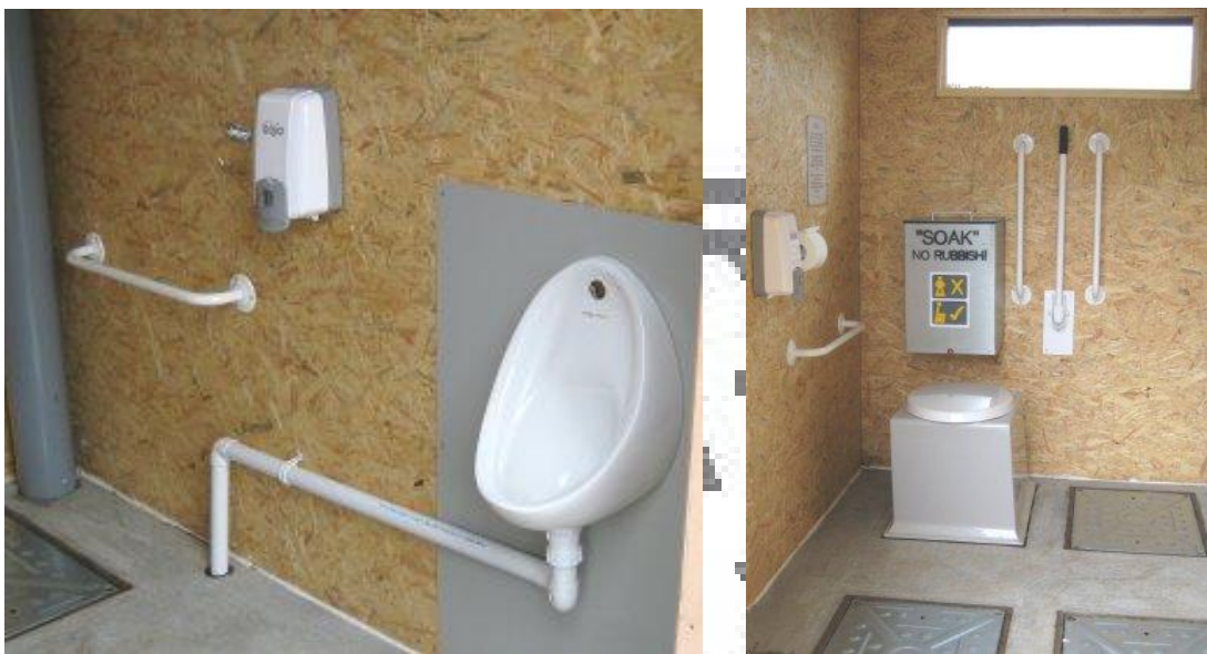
NB The grab rail kit now includes a rail which is fitted vertically to the L of the urinal
